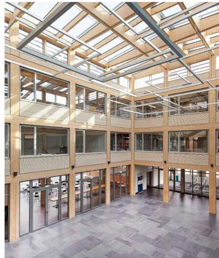
Timber-concrete hybrid building that can be extended in stages with a timber frame curtain wall façade.
