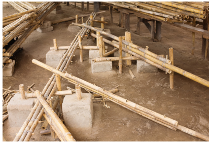
B11 Bamboo workshop: bamboo used to build load-bearing trusses used in roof construction (Photo: Paula Holtz)
