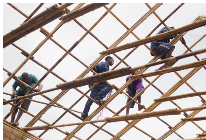
B14 Mounting roof battens (Photo: Paula Holtz)
