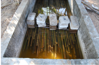
B07 Bamboo laid horizontally for treatment with Borax salt (Photo: Roswag Architekten)
