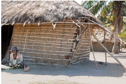
A04 The average lifespan of a traditional house is around five to eight years. Rising damp, termites and leaking roofs all gradually destroy the structures (Photo: Roswag Architekten)
