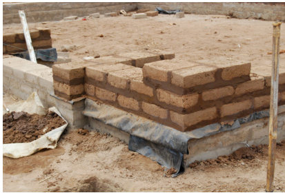
B04 Cement-stabilised earthen block foundation; horizontal damp-proof course; earthen blocks (Photo: Roswag Architekten)
