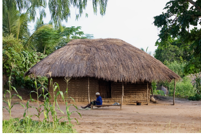
A02 Traditional hut constructed of wood, bamboo and earth using wattle-and-daub technique; grass roof (Photo: Paula Holtz)
