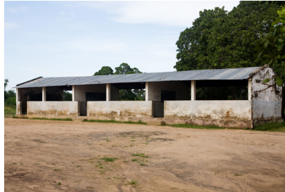
A05 Government-constructed school made of concrete, steel and tin (Photo: Paula Holtz)
