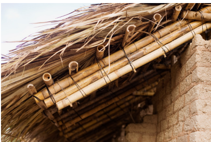
B16 Close-up view of bamboo truss and palm thatch (Photo: Paula Holtz)
