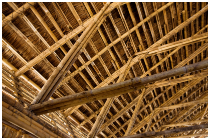
B33 Standard school type in Nacaramo / View of roof construction (Photo: Paula Holtz)
