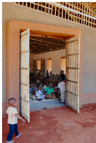
B22 25 de Junho pilot project / View of classroom entrance from outside (Photo: Roswag Architekten)
