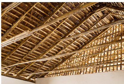
B25 25 de Junho pilot project / Bamboo roof construction (Photo: Paula Holtz)
