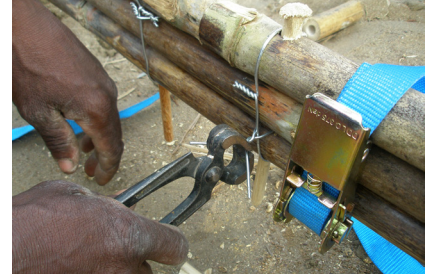
B09 Joints formed on triple-layer bamboo beams using bamboo rods and wire (Photo: Roswag Architekten)
