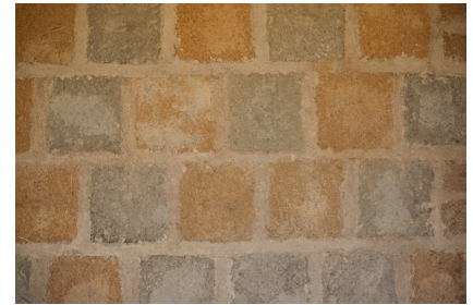
B06 Masonry in simplified school constructions and private homes built by laying traditionally-sized (24 x 24 x 12 cm) earthen blocks upright vertically (Photo: Paula Holtz)
