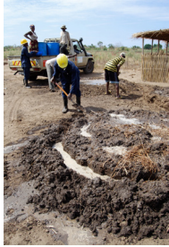
B01 Collecting and mixing earth (Photo: Roswag Architekten)
