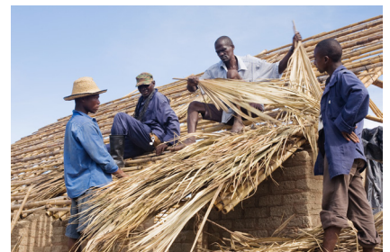
B15 Laying palm-leaf roof thatch (Photo: Paula Holtz)
