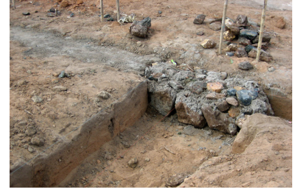
B03 Natural stones used where available to build foundations; cement-stabilised earthen blocks used in other areas (Photo: Roswag Architekten)
