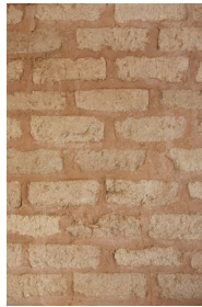
B05 Earthen blocks used in standard school construction type to build 25 cm-thick masonry walls (Photo: Paula Holtz)
