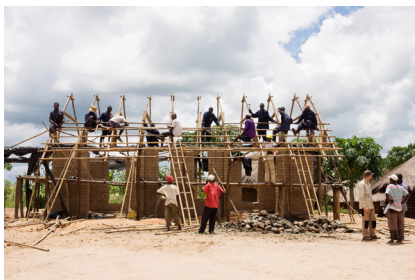
B13 Mounting the roof construction on site (Photo: Paula Holtz)
