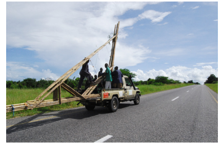
B12 Transportation of the bamboo trusses from the workshop to the site (Photo: Roswag Architekten)
