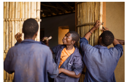
B18 Mounting bamboo doors (Photo: Paula Holtz)
