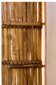
B17 Door lock made of bamboo (Photo: Paula Holtz)
